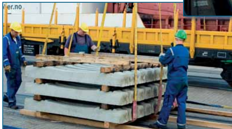
Staff engaged in handling of rails and sleepers
