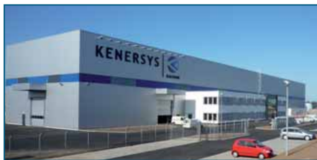
The production facility in Wismar
